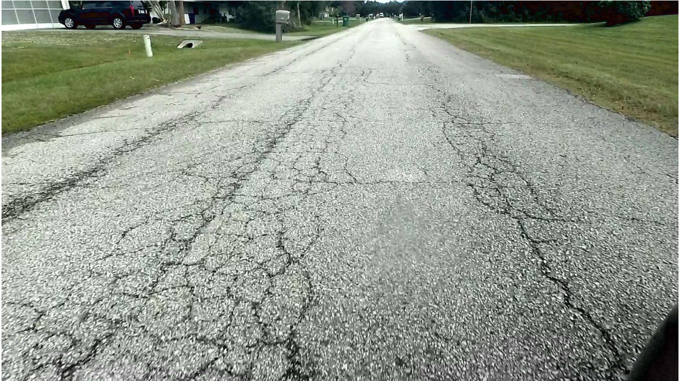
OCEAN COVE ST | SECTION 02 | PCI 28
